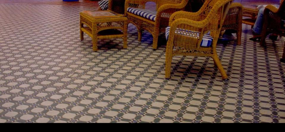
After installation, the floor is grouted with a special polishable grout.
